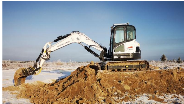
Figure 3. Smart excavation in progress at test site in winter conditions[23]
